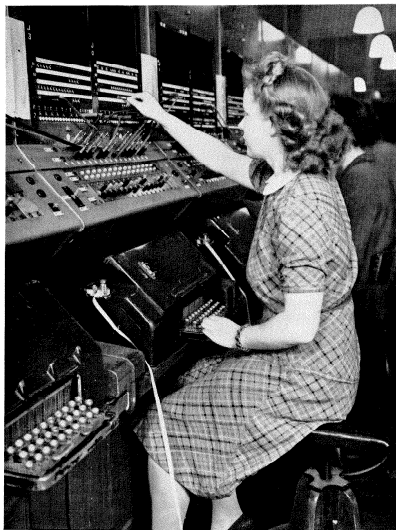
Manual teleprinter switchroom at Manchester, England.
